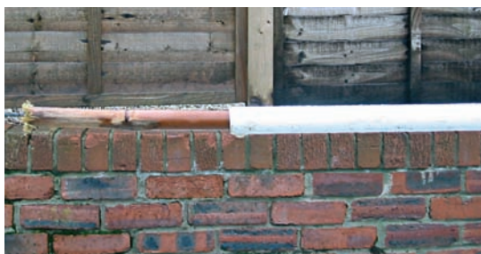
● Fig. 5: When making the spreaders from plastic water pipe, each is reinforced with a suitable bamboo 'cane'. (See text for more details).
